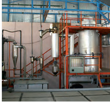
100 kW gasification system for power
