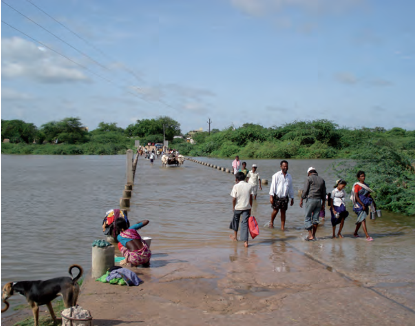
Underwater bridge for crossing a natural drainage channel after rais KC Canal irrigation system
