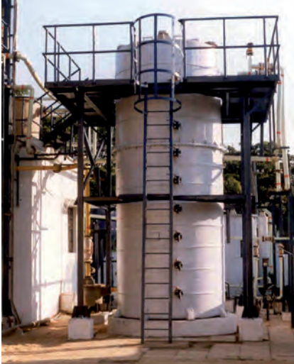
Pilot UASB Reactor at CLRI, Chennai
